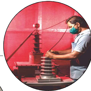
High Voltage Lab upto 200kV
